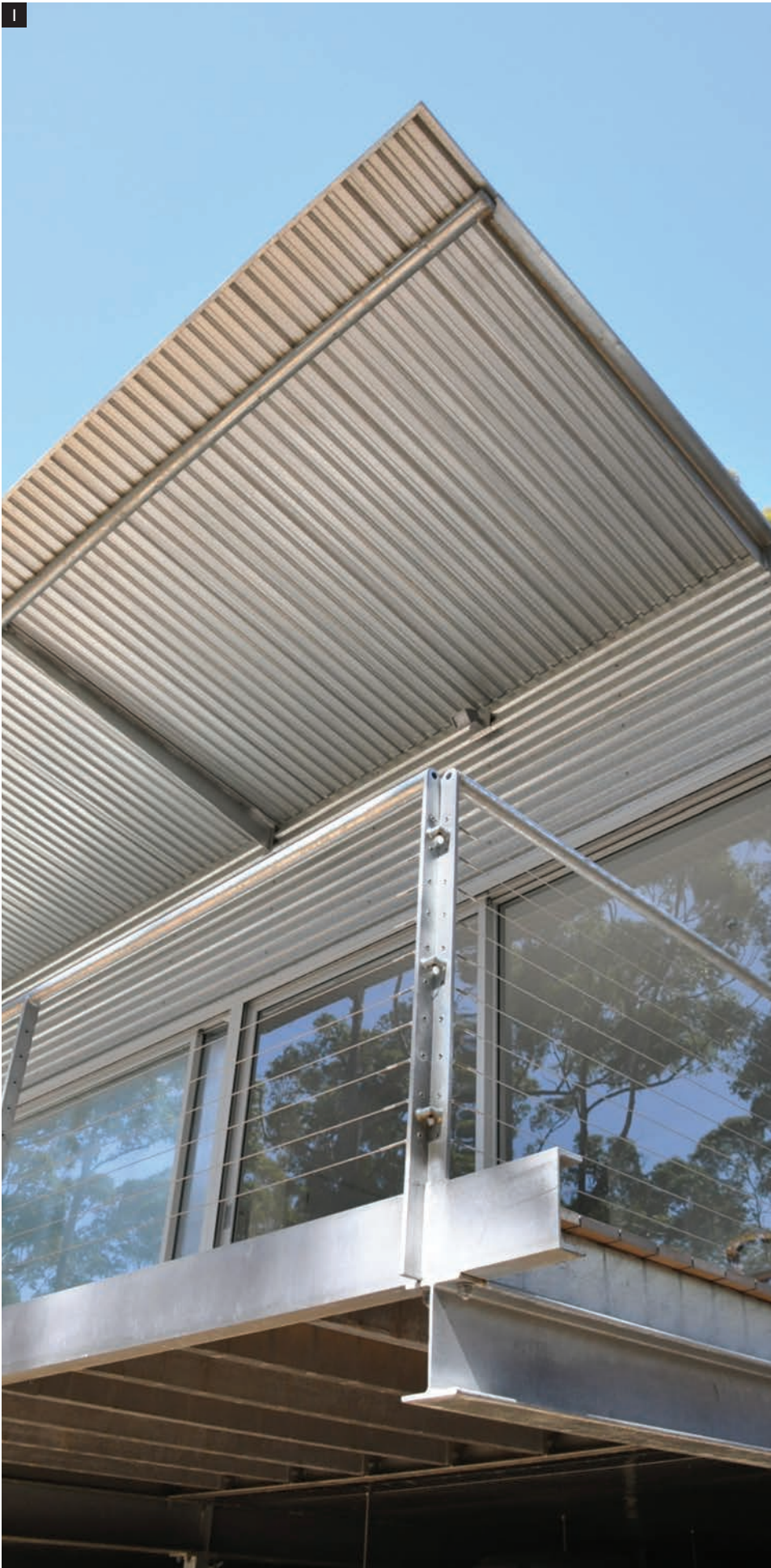
1 The Galvabond and Heritage Galv walls and roof are cost effective bushfire resilient solutions that comply with AS3959 BAL-40. They also weather to a non-reflective texture (unlike Zinalume) and match the granite outcrops and Karri tree trunks
