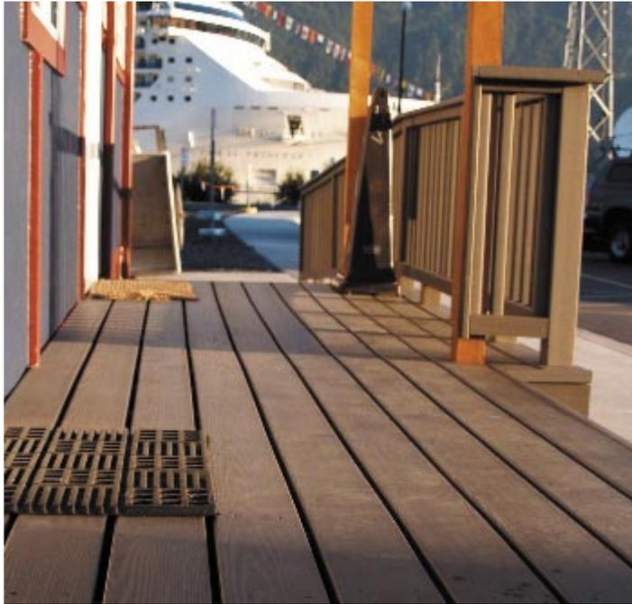
using fibre glass along with wood). Each wood fibre used in composite products has its own characteristics is term rate or tannin bleed (this will leave brown marks on the surface after the first wetting), and durability. The wood fibre is commonly reclaimed from furniture manufacturing (or similar) factories for the use in these products.
