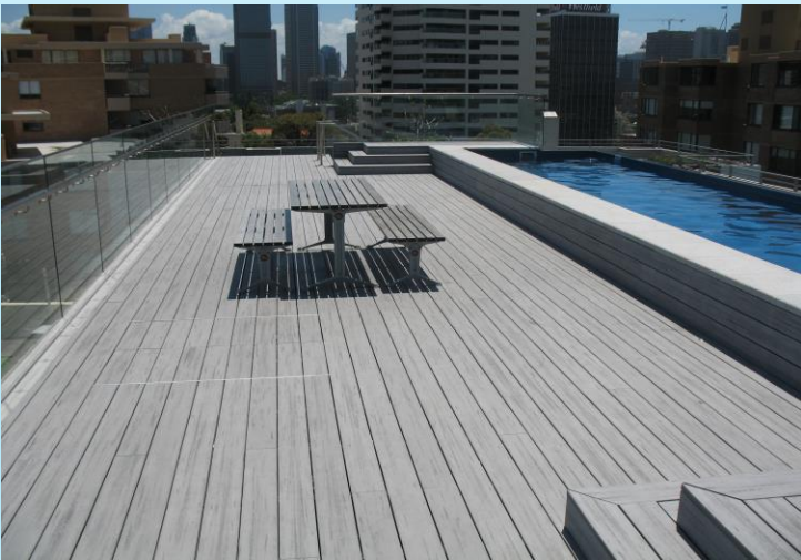
SG 137 Roof Top Pool Darlinghurst
